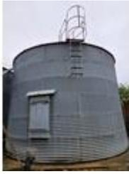
**112.** 50 tonne galvanized grain silo
